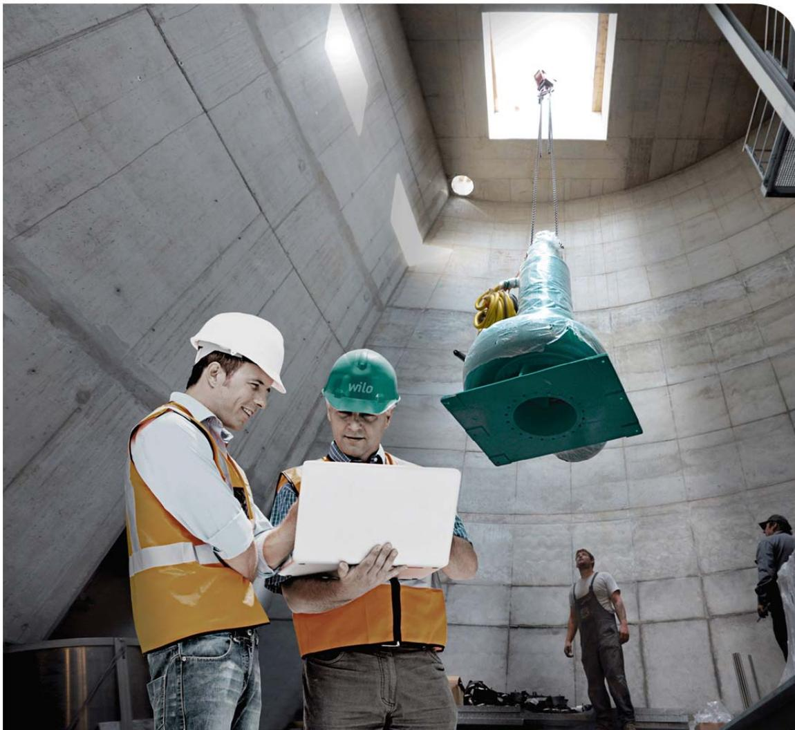
FA 08.64E - 4 pole, 1740 RPM, Non-clog Vane Type
