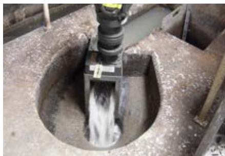
Wet Application 3-HYDRO-C
